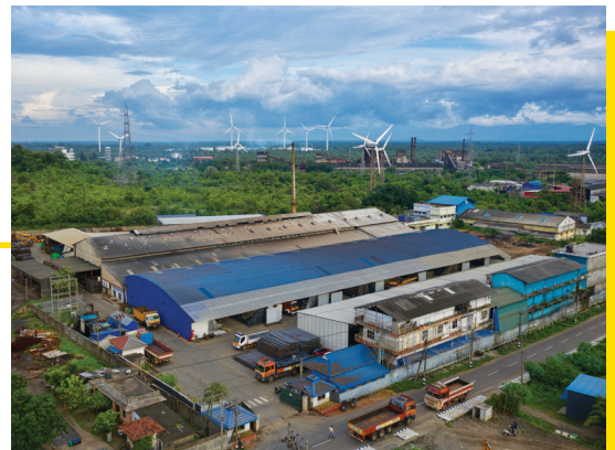
ENVIRONMENT-FRIENDLY PRODUCTION TO CONTROL POLLUTION AND REDUCE WASTAGE
